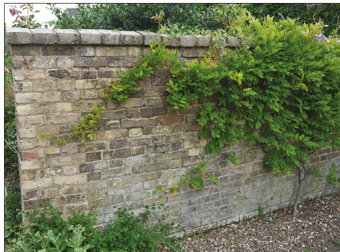
Figure 44: Lodge Close Wall.
